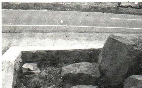
Figura III.4. Alcantarilla Azolvada
